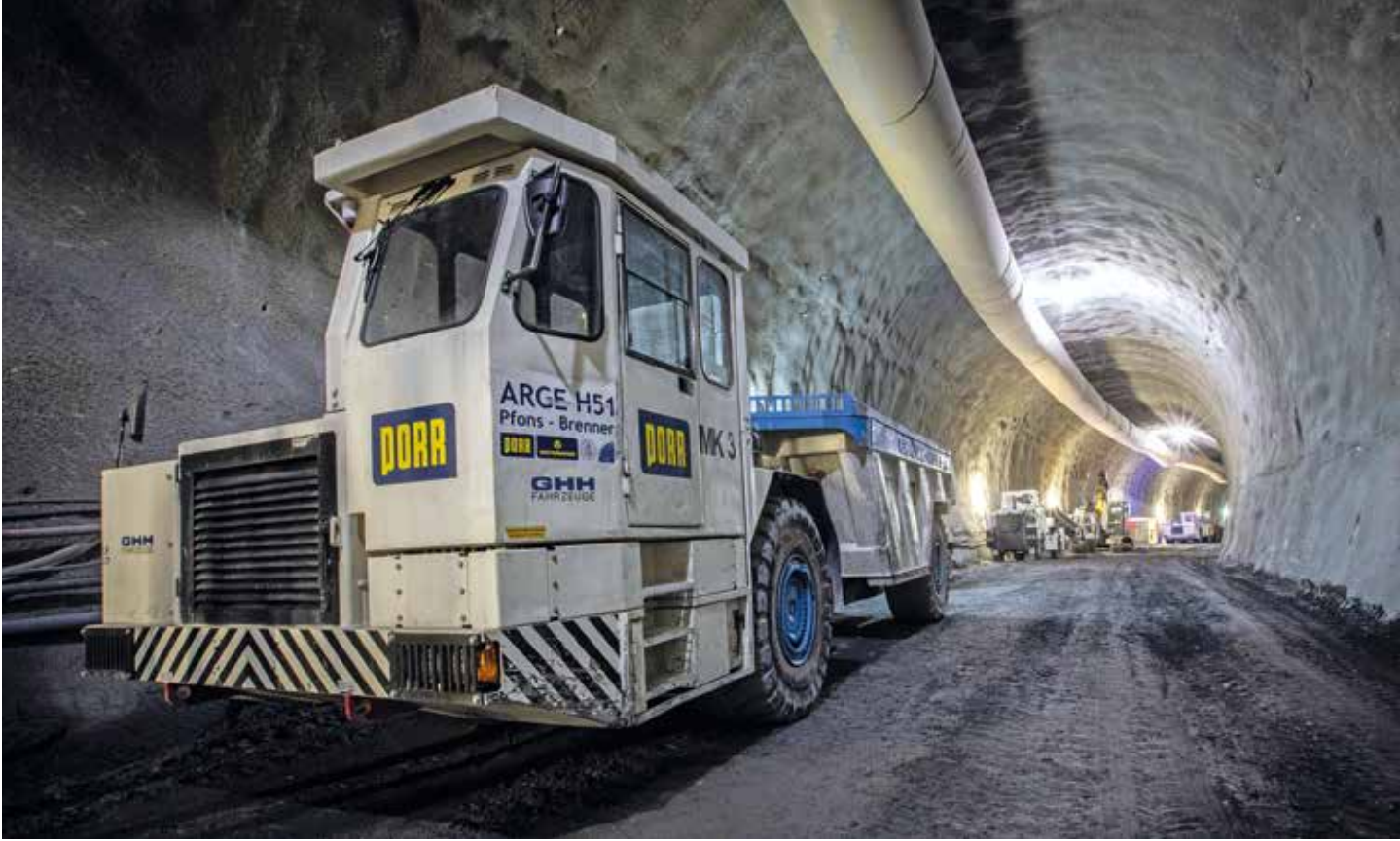
Dump truck, Brenner Base Tunnel
