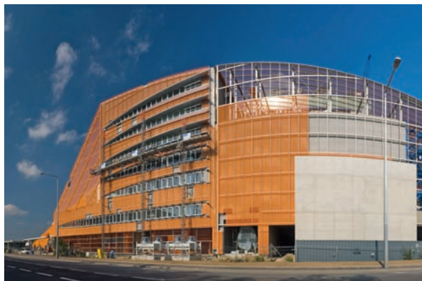
Pfaffenau waste incineration plant
