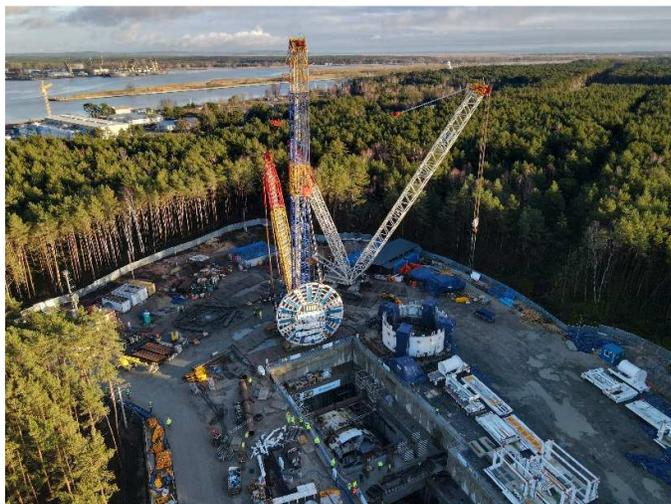
*TBM shield assembly in Świnoujście (© PORR)*
